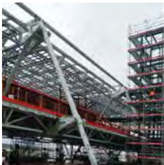
MARTIFER METALLIC CONSTRUCTIONS
