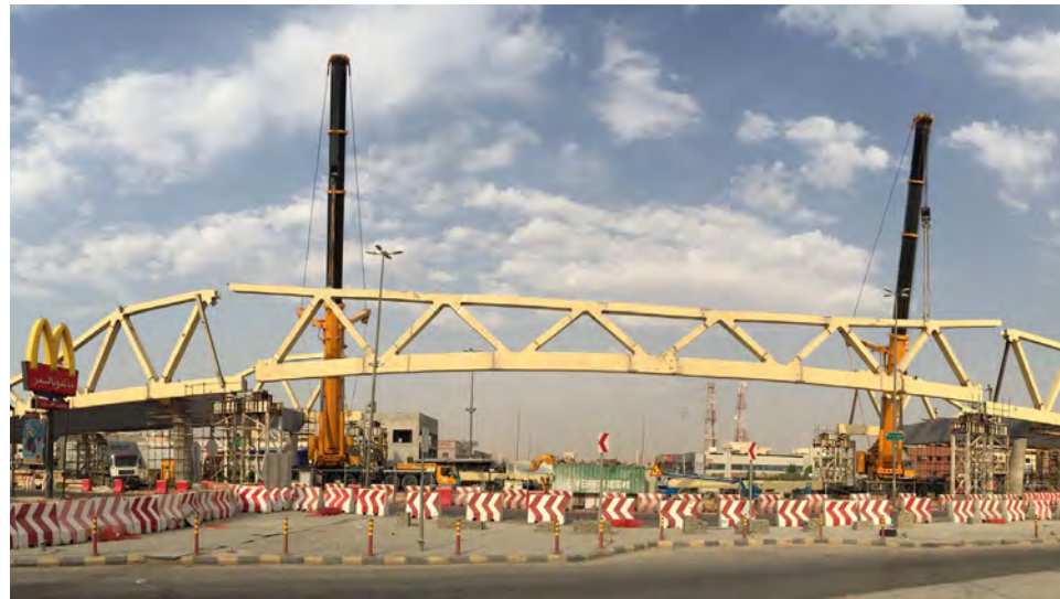
Abi Bakr Bridge
