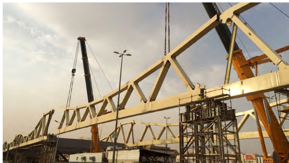
Abi Bakr Bridge
